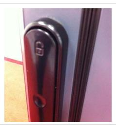
Ensure the 'unlocked' symbol is at the top before opening doors
